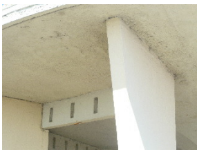
5 Street name: Beach Street Building name: Shelter
